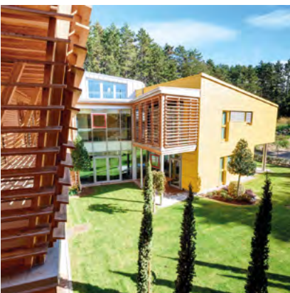
Casa Sebastiano Coredo - Italy
